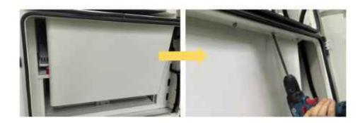
Step 2:Remove the inverter and fix it on the side of the cabinet. Note: The inverter is quite heavy. Be careful not to bump it. Installation must comply with the inverter standards.
